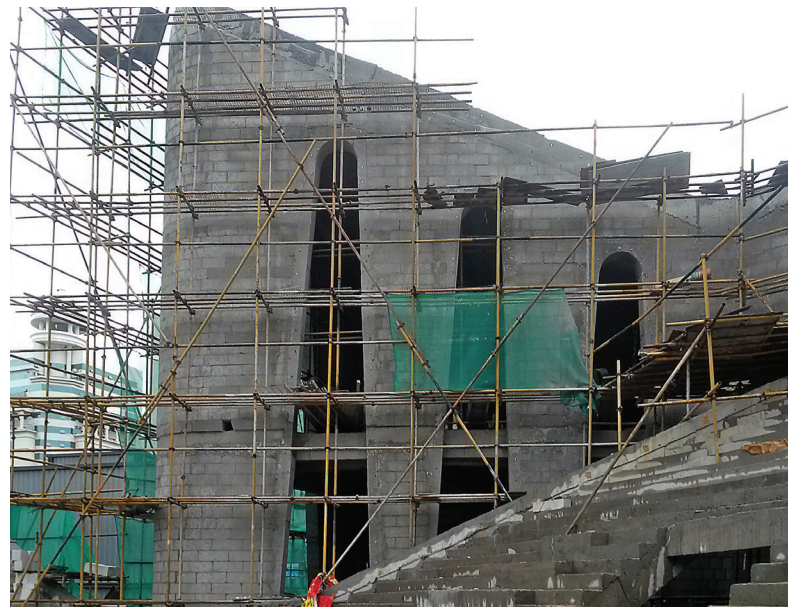
Top left: Peace in the eye of the storm – upper amphitheatre (south-east direction). Top right: First phase of construction with the inner concrete framework being cast. Above: Façade framework filled with aerated concrete blocks. Below: Lower amphitheatre – a space for open-air worship and gatherings.
